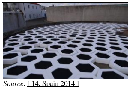
Figure 4.78: Geometrical plastic tiles in a slurry tank
