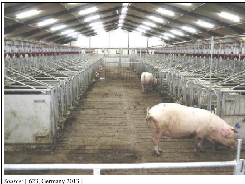
Figure 6.4: Gestating sow room of the near-zero-emission pig housing system showing the 'roof-ceiling' construction principle
