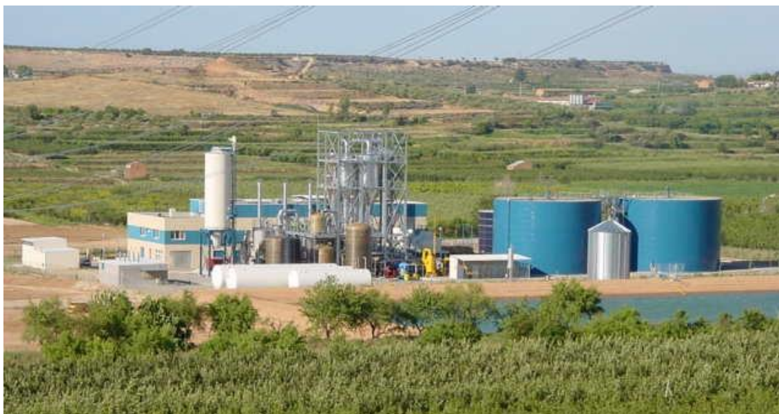
Picture E.13: General view of the plant
