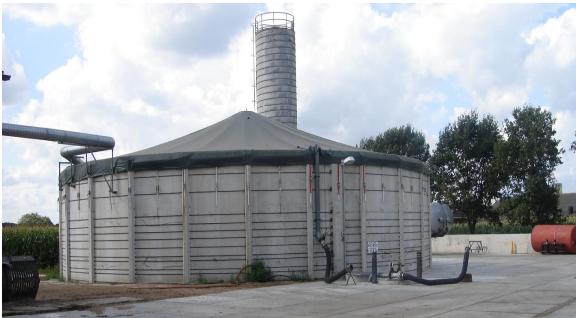
Picture C.3: Slurry tank for reception of slurry.
