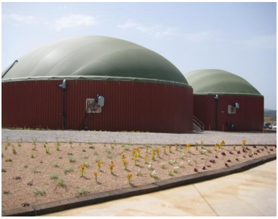
Picture G.4: Anarobic digesters
