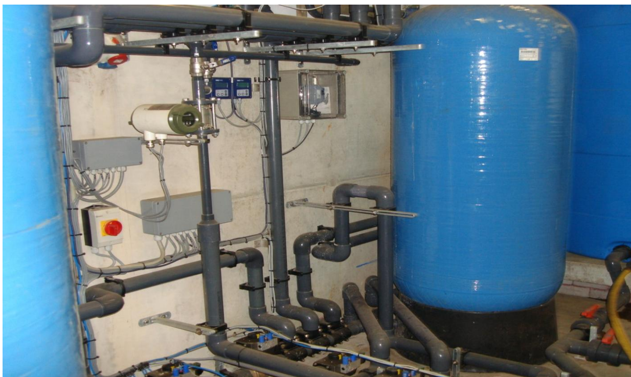
Picture C.9: The liquid fraction is de-mineralised in the final step before being deposited in the nature.
