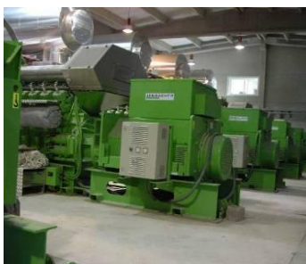
Picture E.8: CHP engines
