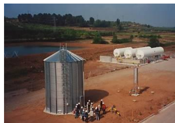
Picture E.3: Gas holder and flare
