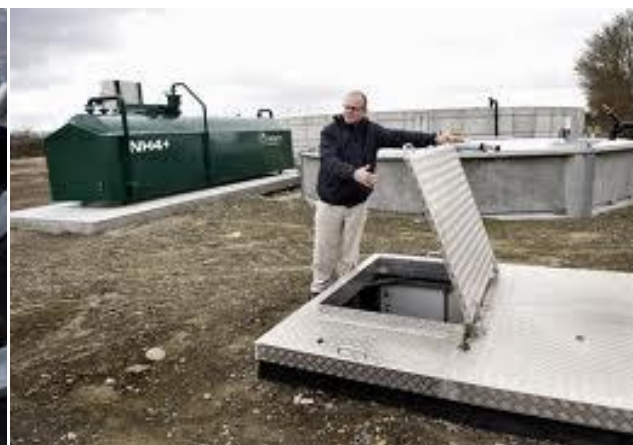
Picture B.3: From left: Acid tank, process tank and a look in the valve pit.
