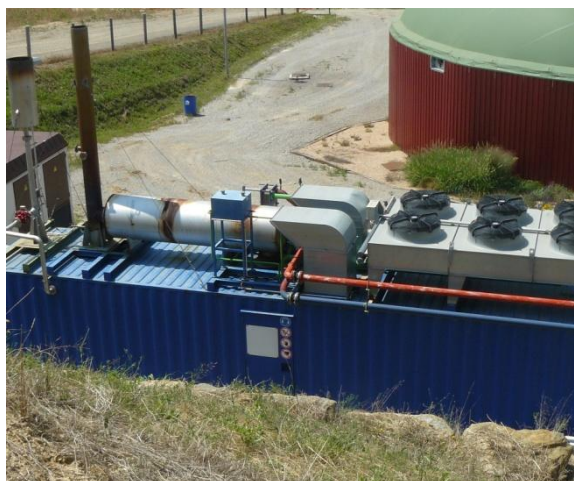
Picture G.7: Container with CHP engine
